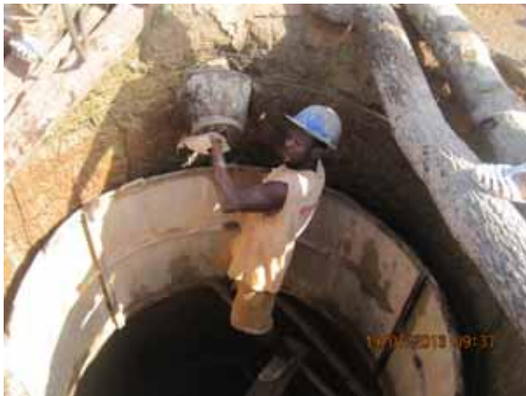
Brunnenbau in Toumoudoto
